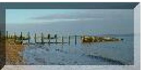
As the Groynes are made of wood they do tend to rot and need to be replaced regularly.
