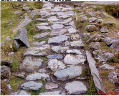
2) Aggregate –Small Particles of hard material usually loca I stone laid on the existing surface, the slope must be less than 15 degrees this is a lot less labour intensive than pitching therefore is much cheaper.
