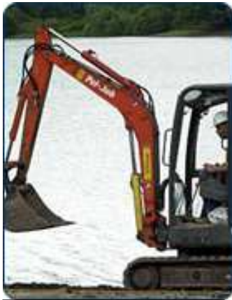
Although there is heavy construction it is carefully managed.
